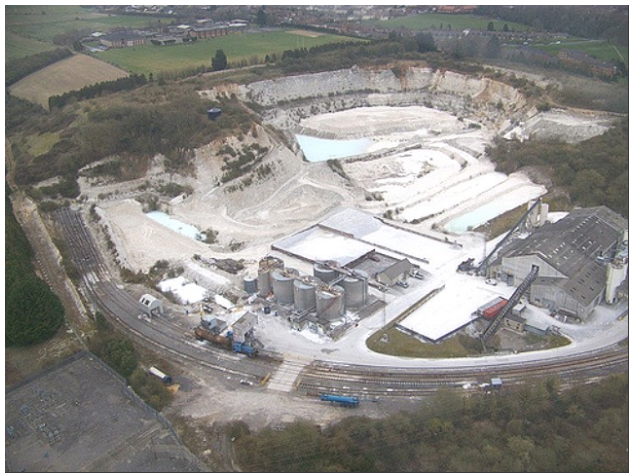
Quarry in 2009, before closure and demolition of buildings
