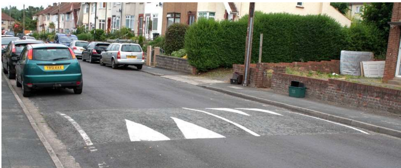
Figure 18; Example of a speed hump (note position of parked cars)
