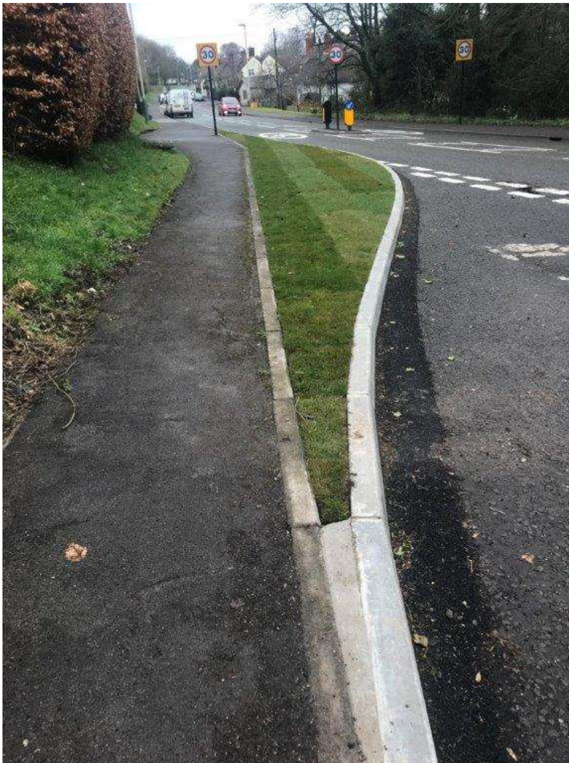
Figure 13; Example of road narrowing using hard feature
