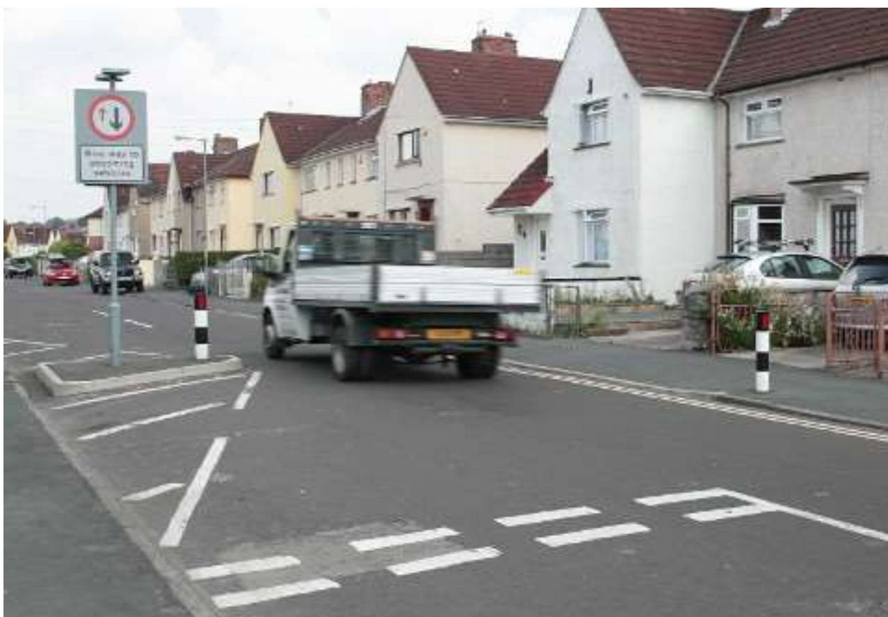
Figure 16; Example of chicane (note position of driveways). Note the position of the bollard and also the gap left for drainage; a wider gap can also be left for cycles.
