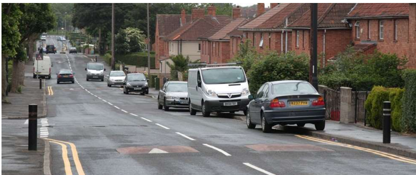
Figure 20; Example of speed cushions (note position of bollards adjacent to carriageway; note position of double yellow lines; note proximity to junction)
