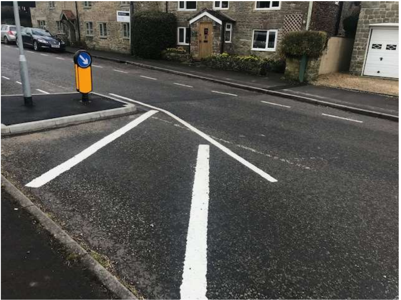
Figure 14; Example of build out of the kind to produce chicanes (here used instead to provide a longer pinch point including parking). Note the position of the bollard and also the gap left for drainage; a wider gap can also be left for cycles.
