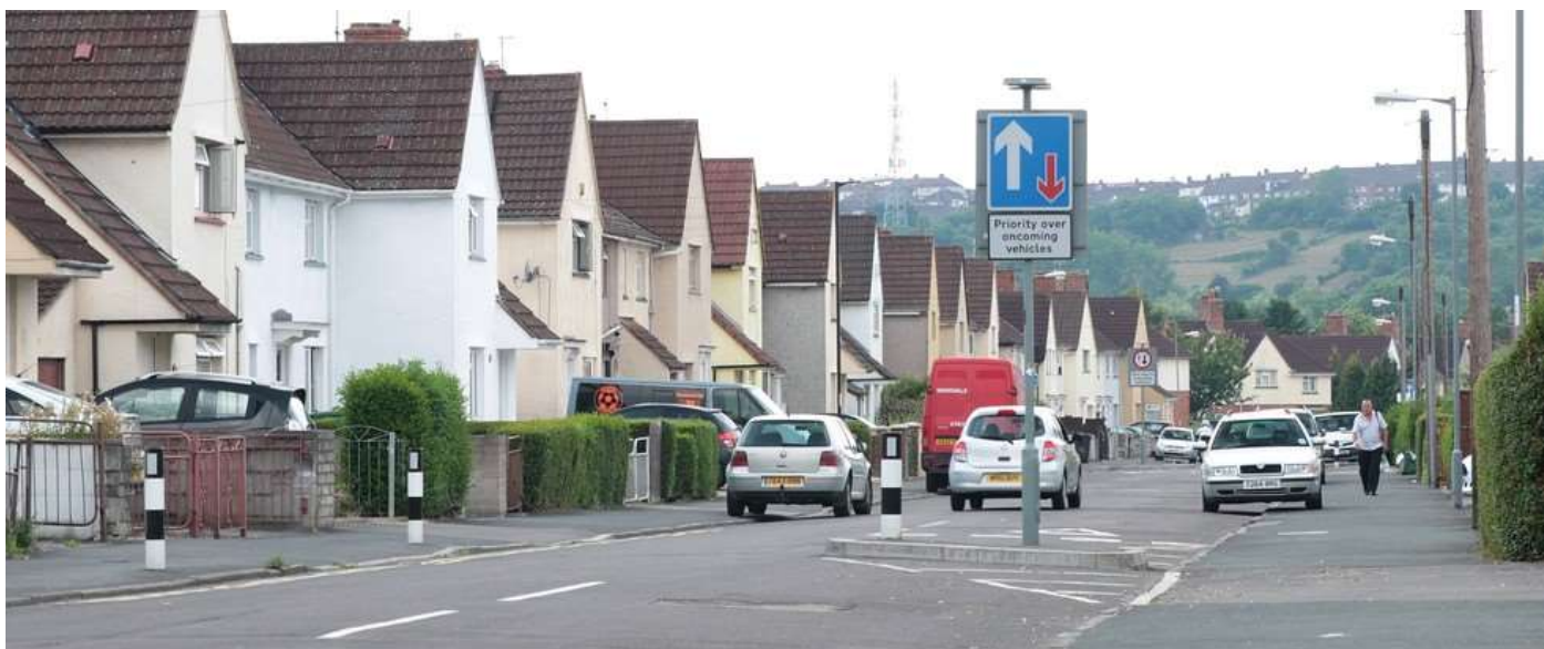
Figure 17; Example of chicane (note position of driveways). Note the position of the bollard and also the gap left for drainage; a wider gap can also be left for cycles.
