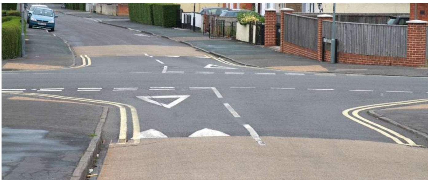
Figure 19; Example of speed table at a four-way junction
