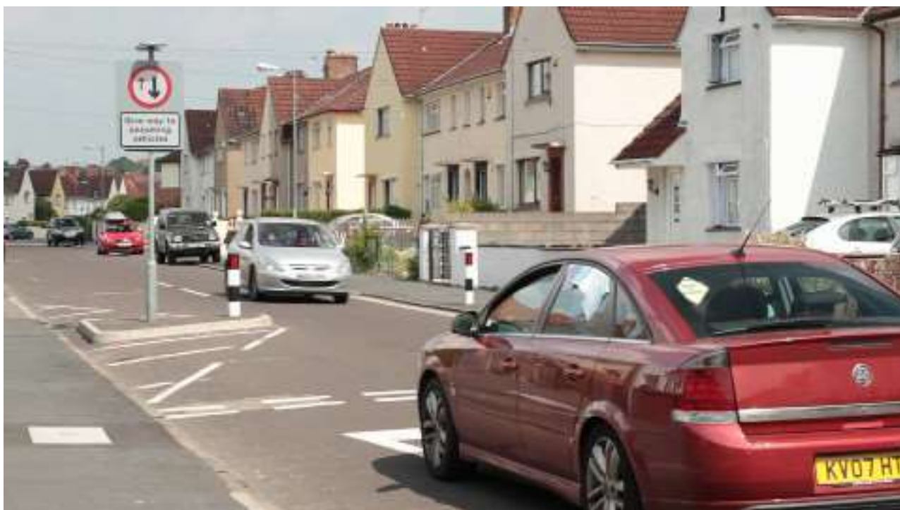
Figure 15; Example of chicane (note position of driveways). Note the position of the bollard and also the gap left for drainage; a wider gap can also be left for cycles.
